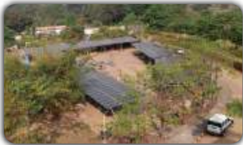
Solar Carport Plant
